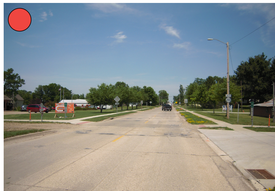
Highway 17 and High Trestle Trail Intersection. Source: Nate Schlorholtz
